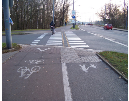
Most fatalities and injuries to pedestrians and cyclists occur in urban areas. Proper infrastructure design can help to reduce number of KSIs 2 . Photo source: cs.Štů
